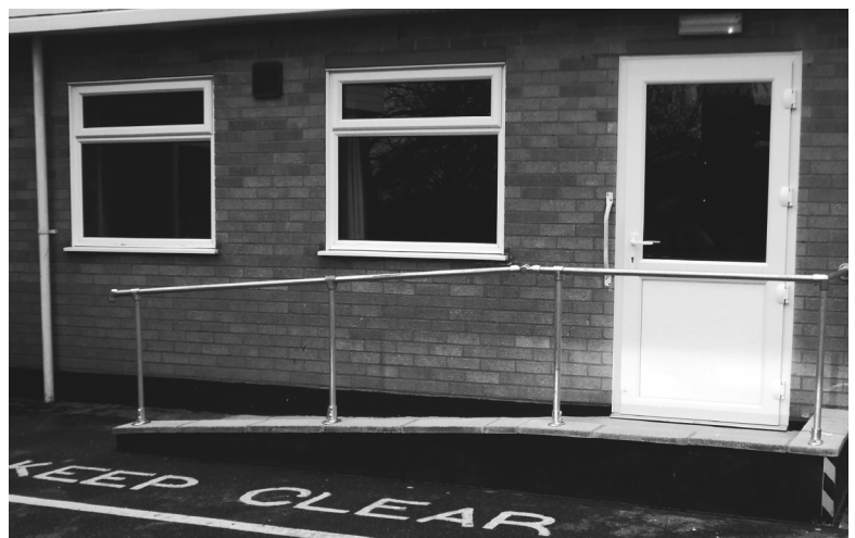
The new disabled access ramp to the Post Office in the Community Centre.
